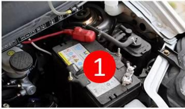
1. BATTERY of car is install in the engine room
